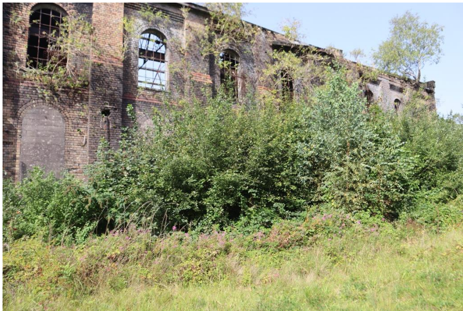
Figure 4.13. H7 along the building
