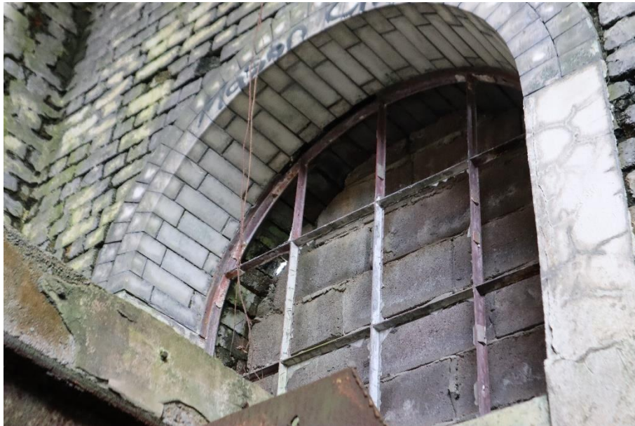
Figure 4.18. Limited gaps around windows
