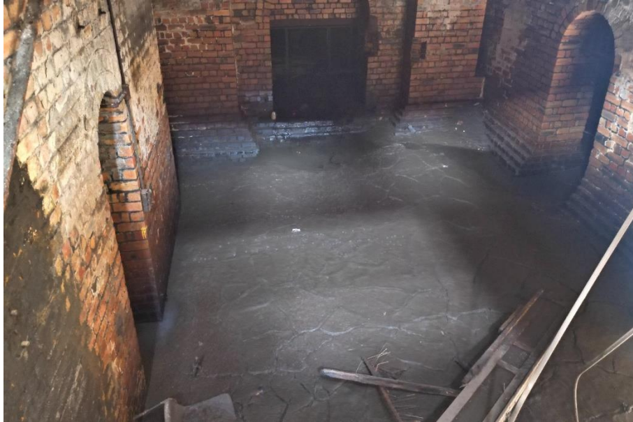
Figure 4.12. Sub-floor of H6
