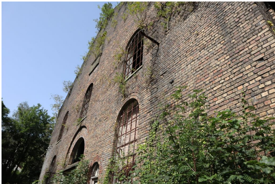
Figure 4.9. Southern gable of H6
