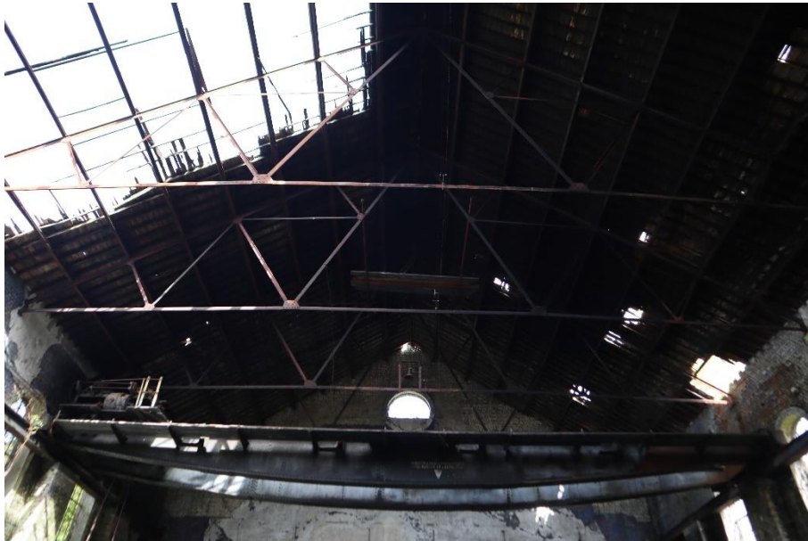
Figure 4.11. Showing the metal trusses supporting the roof in H6
