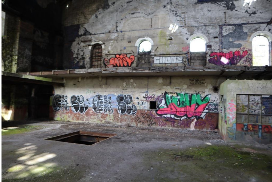
Figure 4.10. Typical view inside H6
