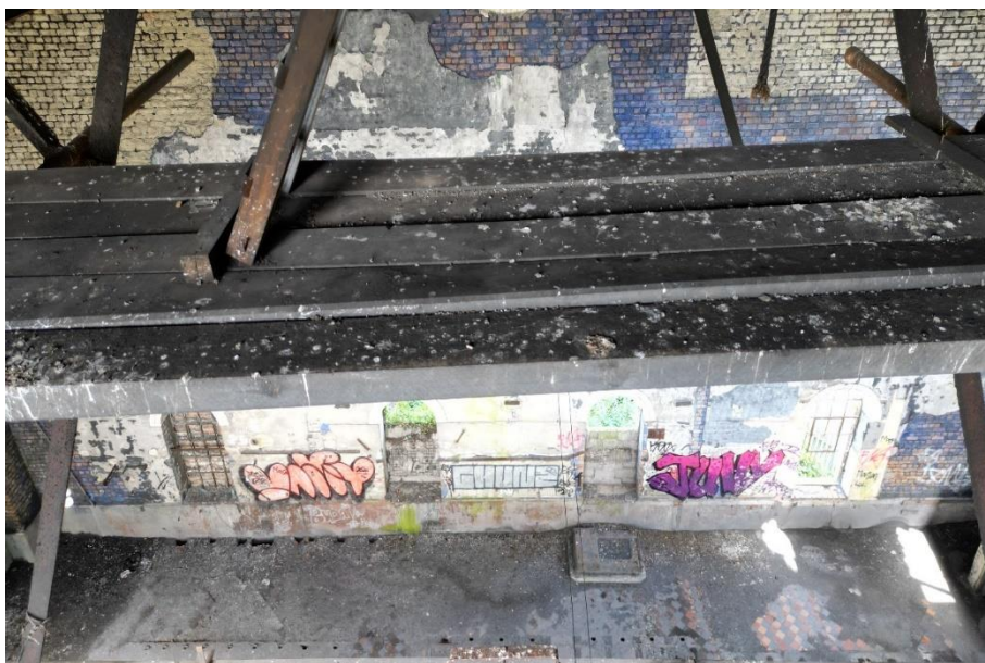
Figure 4.21. Perching platform near roof of building
