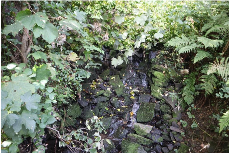
Figure 4.16. Stream coming down from culvert under road
