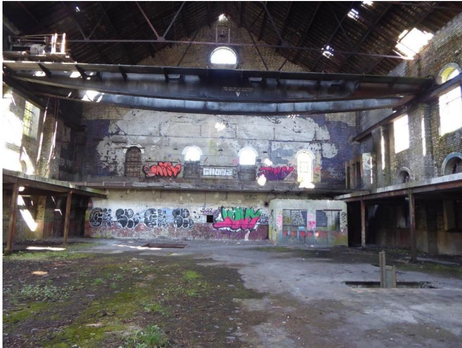
Figure 11 Interior looking north showing the overhead crane
