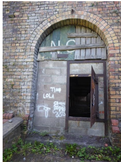
Figure 8 Entrance near north-east corner
