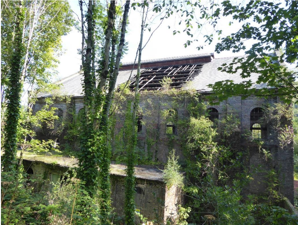
Figure 6 West elevation as seen from Llwynypia Road
